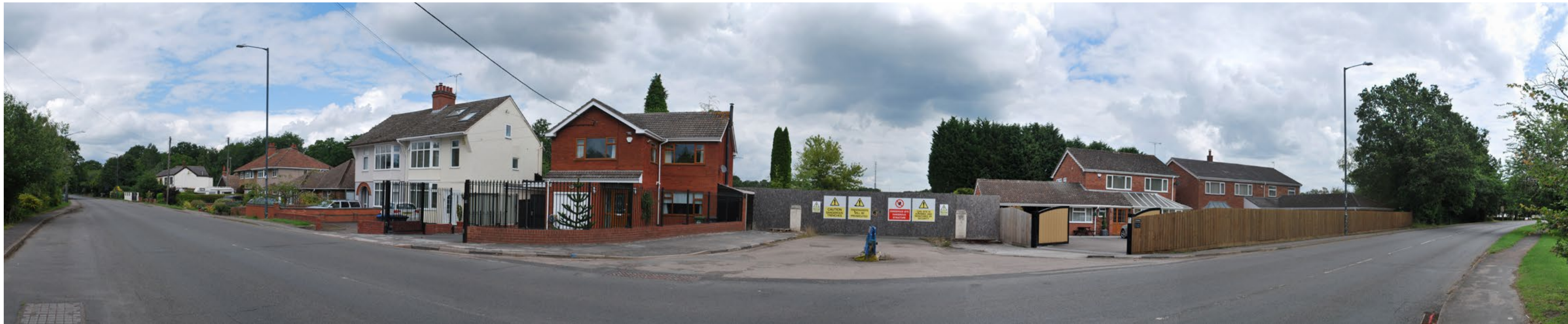
Appeal Site Context Photograph 1: View looking north-west from Rugby Road (A428).
