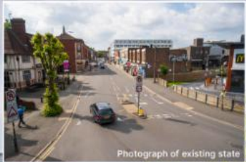
Photograph of existing state
