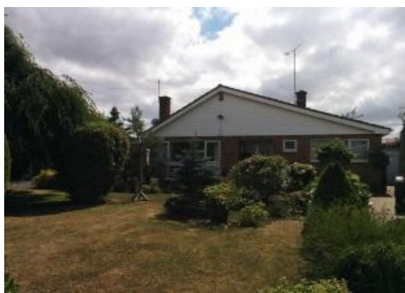
Bungalow with closed gable end facing the road
