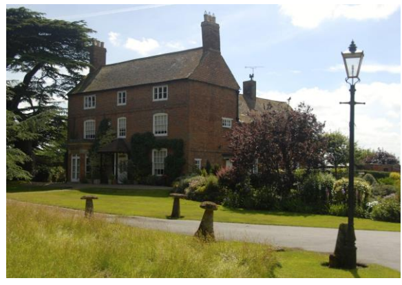
2. Manor Farmhouse (Grade II)
