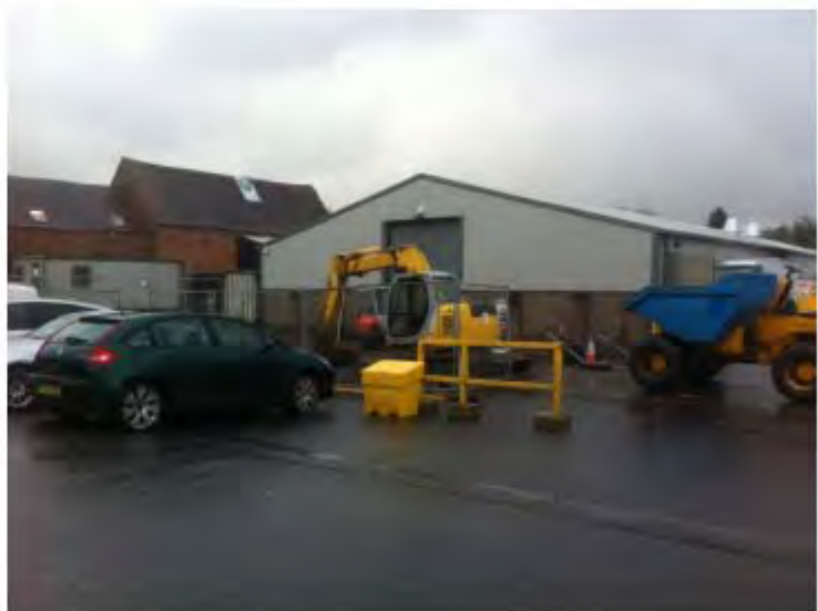
Fig 5. Existing Production Facility (Extension under construction)
