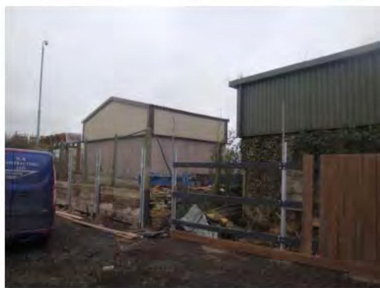
Fig 7. Stonemarket Adjacent Buildings (New fencing is now complete)
