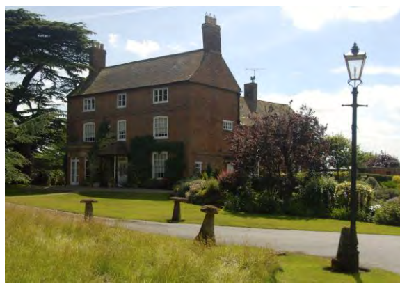
2. Manor Farmhouse (Grade II)
