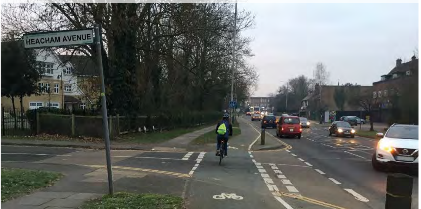
Figure 10.16: Partial set back, marked priority crossing, Hillingdon
