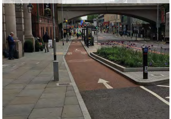
Figure 9.4: Cycle lane to cycle track transition
