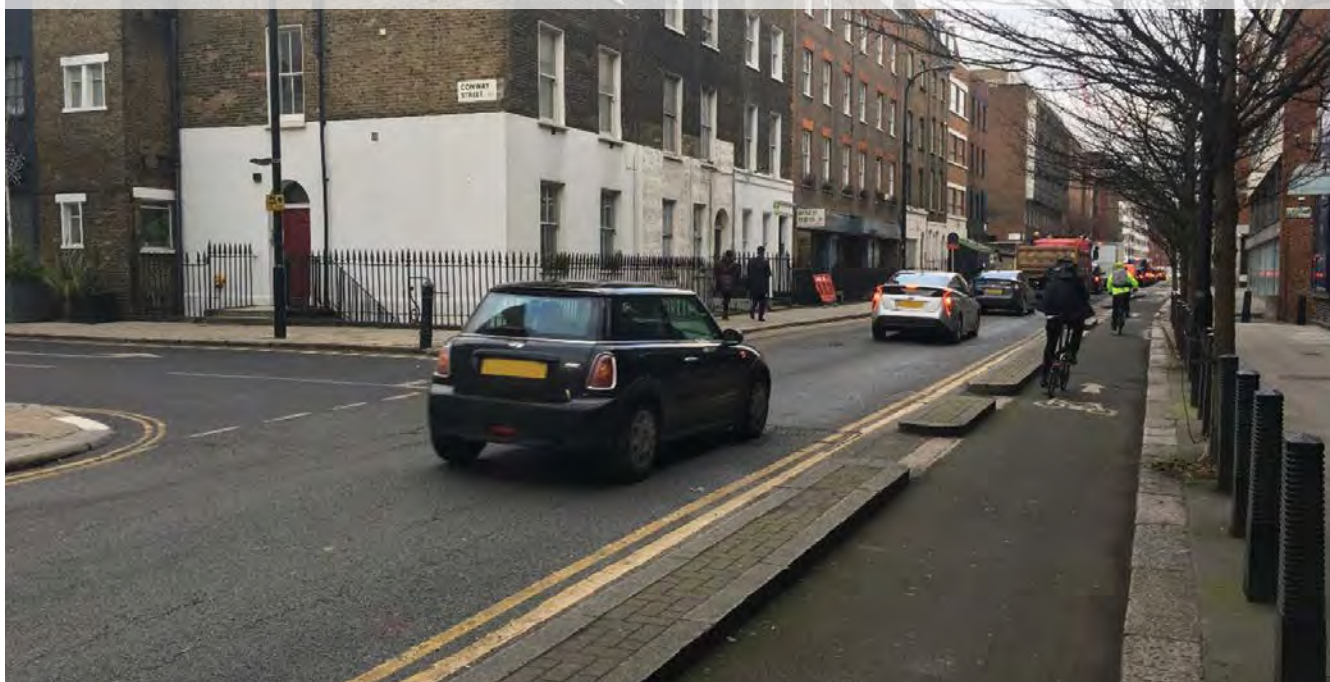
Figure 6.9: Carriageway level cycle track with gaps in buffer strip to access side road – Camden
