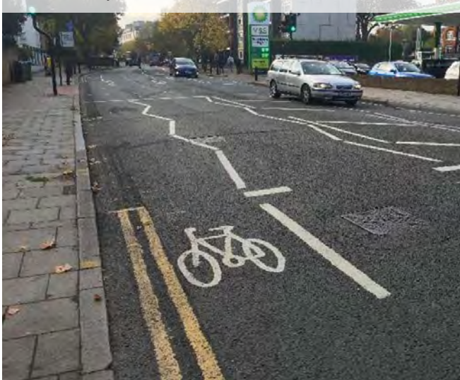
Figure 6.19: Zig-zag markings placed away from the kerb to continue cycle lane, Greenwich
