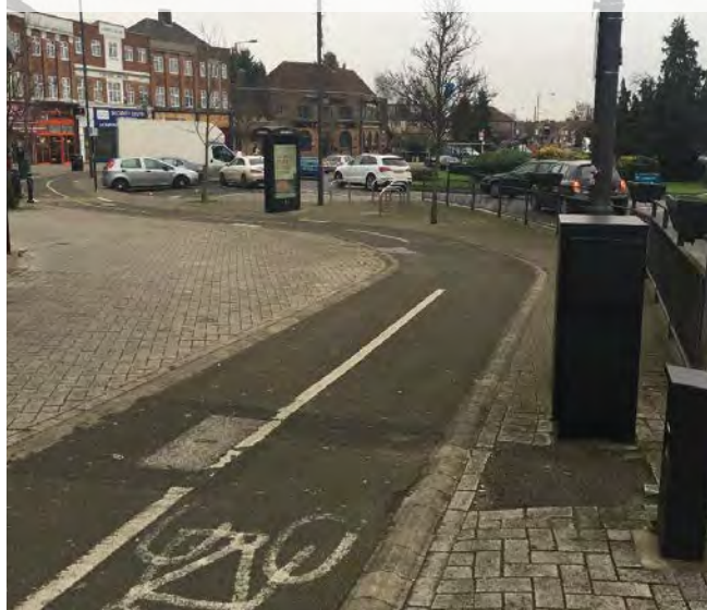
Figure 10.36: Footway-level cycle track around large roundabout, Harrow
