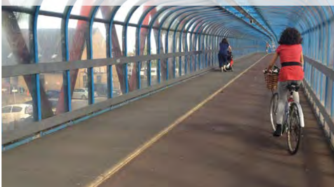
Figure 10.50: Covered pedestrian/cycle bridge across railway tracks, Cambridge
