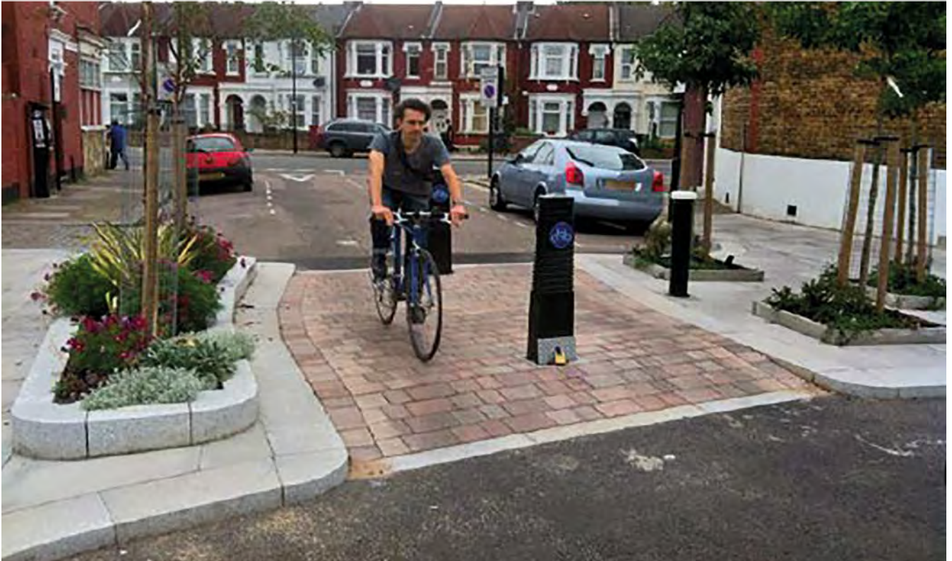
Figure 7.1: Simple modal filters can reduce through traffic while retaining cycle and pedestrian access. The central position enables kerbside car parking to be provided without blocking the facility, and the lockable bollard enables emergency access, Haringey.
