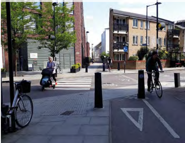
Figure 10.7: Parallel crossing, Hackney
