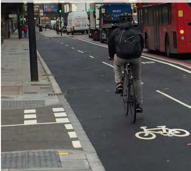
Figure 7.10: Tight kerb radii at residential side street
