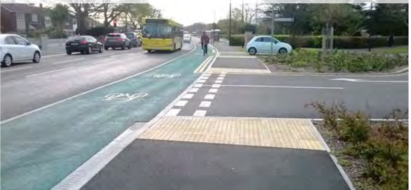
Figure 10.17: No setback crossing with design priority,– Bournemouth
