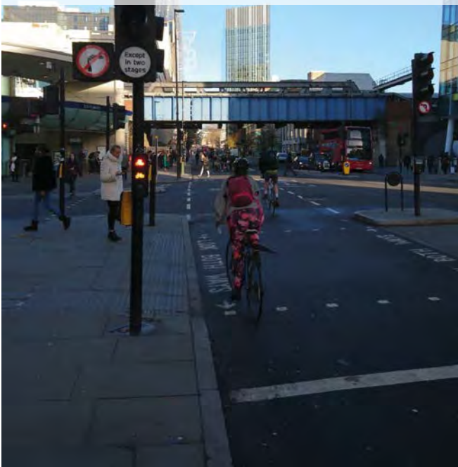
Figure 10.21: A LLCS used as a repeater beneath an HLCS (London)
