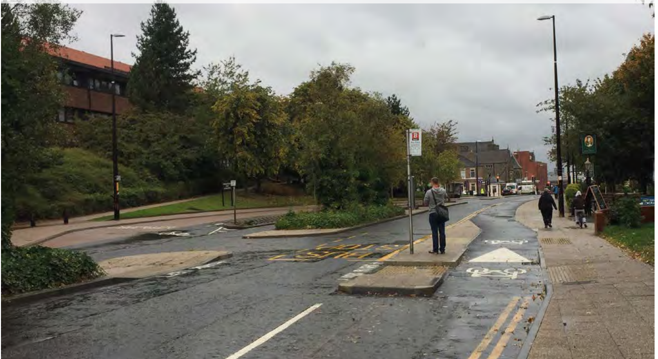
Figure 9.3: Cycle track joins cycle lane after bus stop, Gateshead
