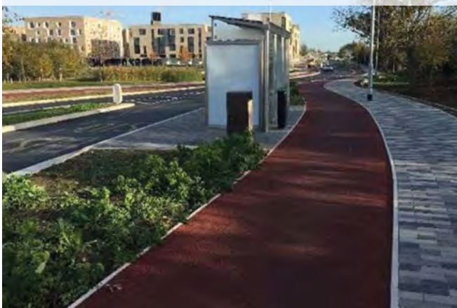
Figure 14.4: One way footway level cycle track past bus stop, North-West Cambridge development.
