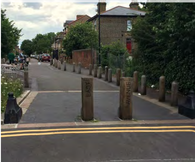
Figure 1.9: Bollards used to create modal filter, preventing through traffic
