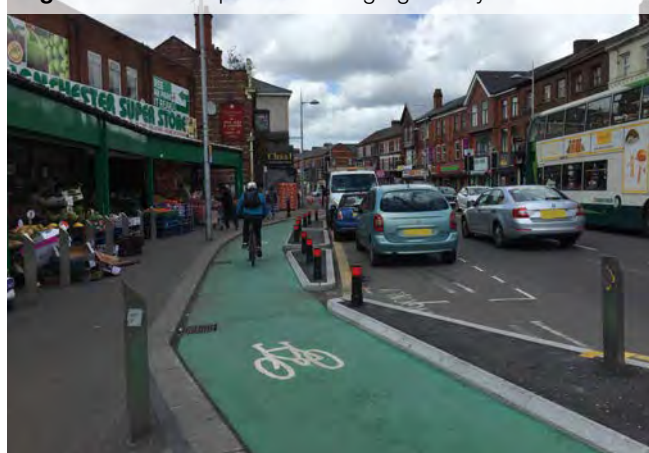
Figure 1.10: Example of kerb-segregated cycle track
