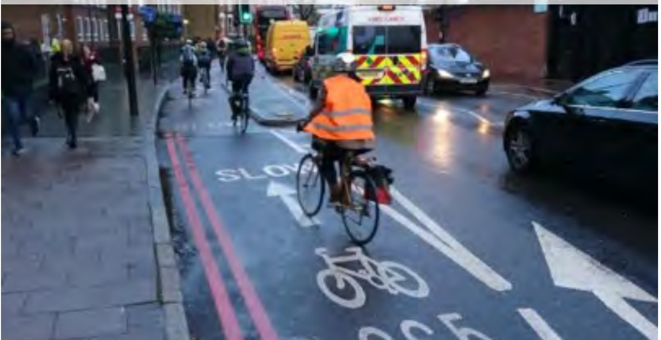
Figure 10.24: Cycle bypass of signals, Oval, London. Cyclists may turn left at the signals onto a shared use path.
