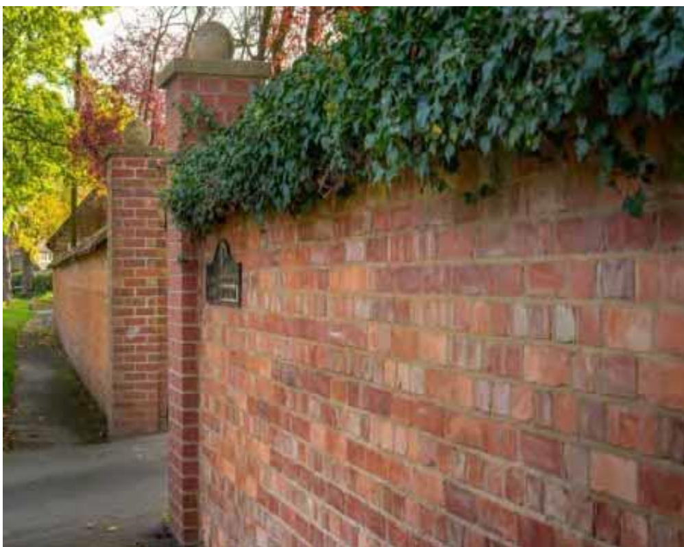
Boundary wall of the Nursing Home facing Main Street
