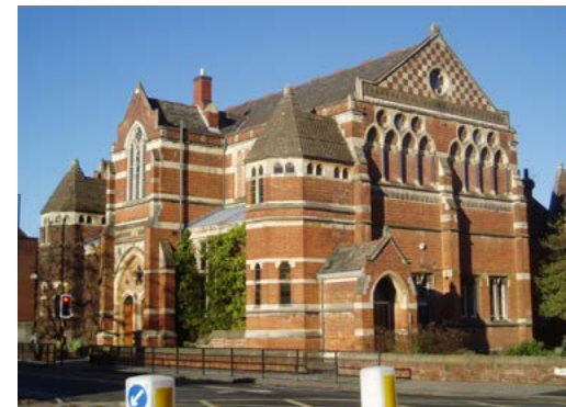
New Big School Building on Lawrence Sheriff Street
