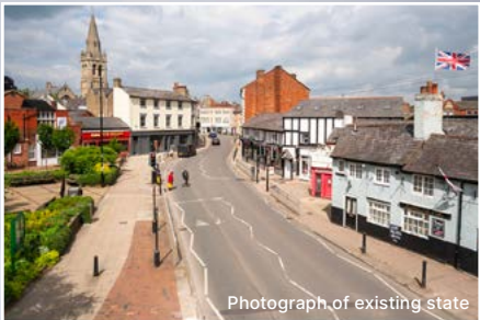
Photograph of existing state
