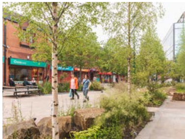
Public Realm SuDs/ Planting areas Hard landscape drains into planting areas Allowing for 1 x 10m 2 every 20m of streetscape.
