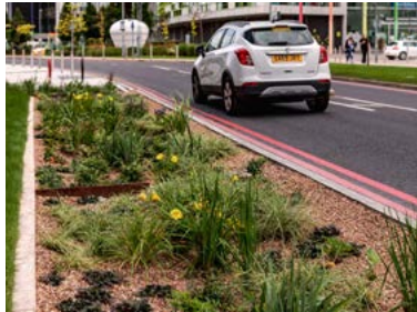
Highway SuDs - The Stitch Allowing for 2 x 10m 2 every 30m of streetscape on either side of the road.
