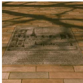
Natural stone paving with bespoke elements that connect the space to its heritage.
