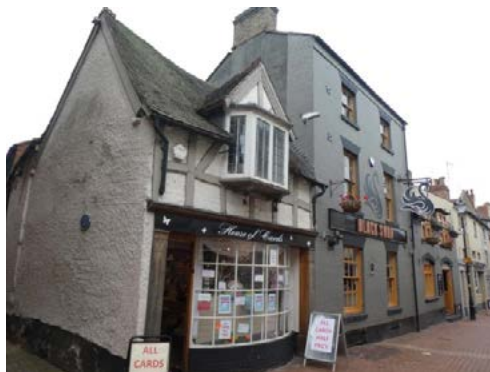
Medieval Building, Chapel Street.
