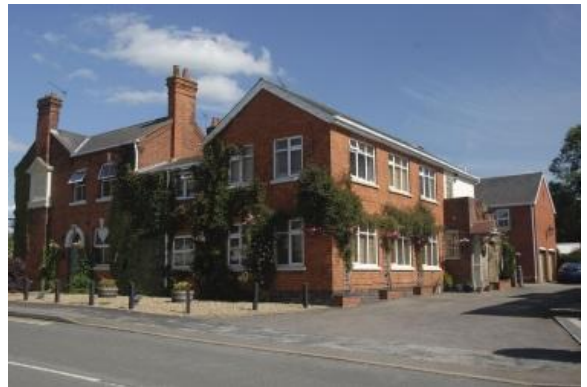
The Four Crosses apartments opposite the bungalows
