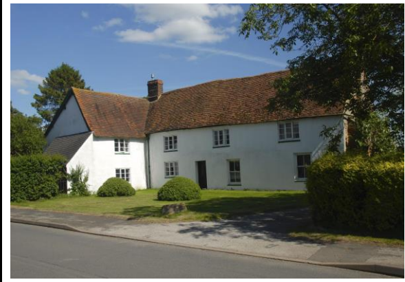
7. Whitehouse Farmhouse (Grade II)
