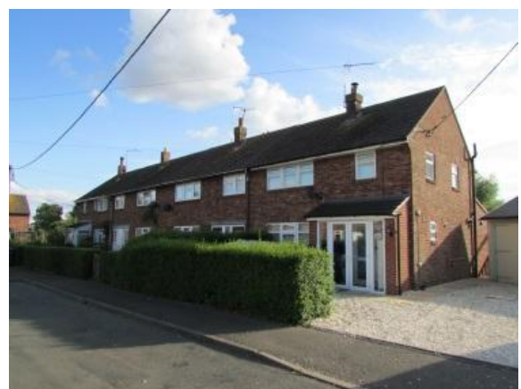
The terrace of four on the west side
