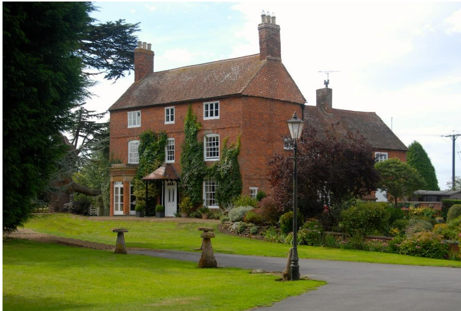
Manor Farmhouse (Grade II)
