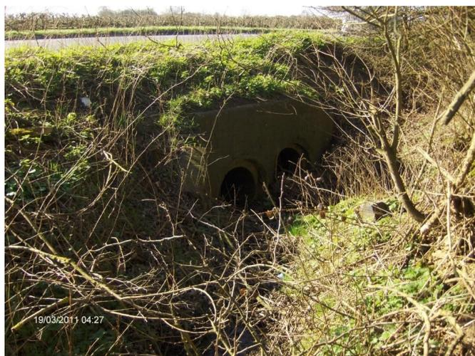
*Partly silted culverts under A45*
