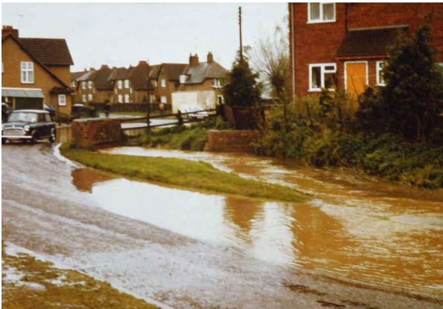
Photograph 3. Brook topping bank at Village Hall Bridge
