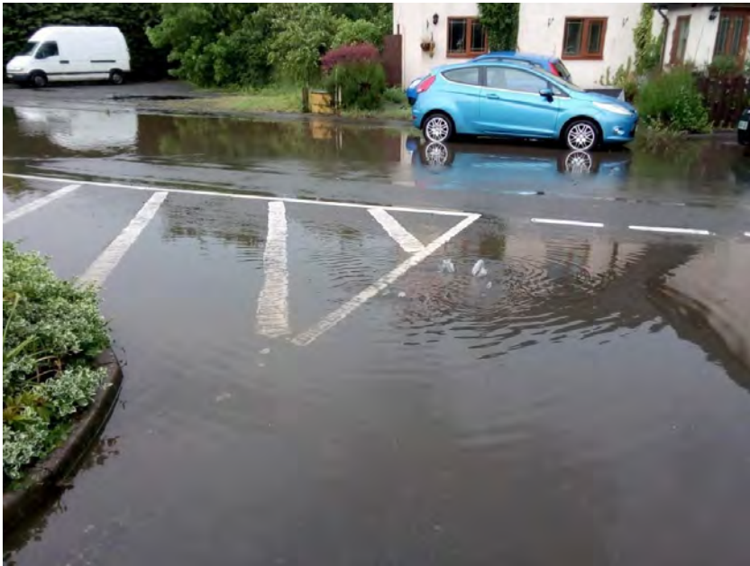
Photograph 11. Flooding on 27 th May 2018 showing sewer refluxing.
