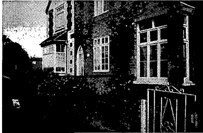
Figure 64 - Featuring an original timber window in a brick bay in the foreground and painted stone dressings to the end of terrace
