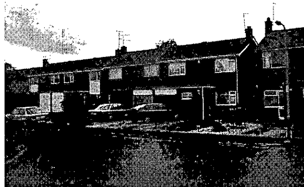
Figure 68 - Newall Close illustrating 1960's semi-detached houses with integral garages
