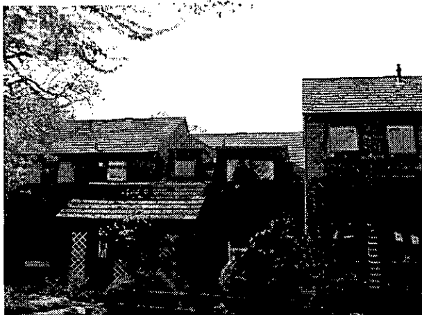
Figure 59 - Staggering the building line, changing the roof level and inserting dormer windows add variety to a uniform style of building
