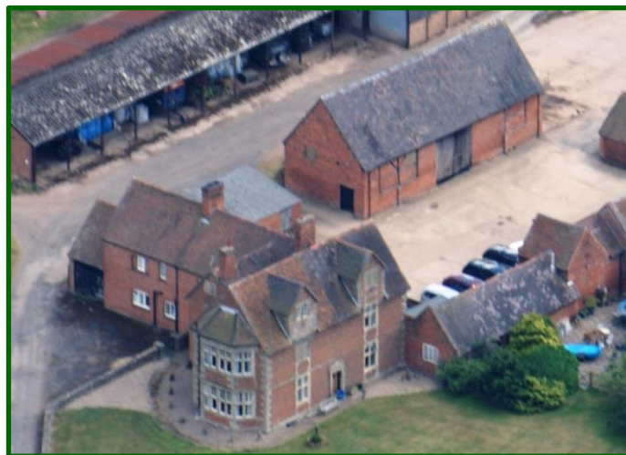
Old Lodge Farmhouse and Barn
