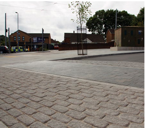
Setts with Asphalt
