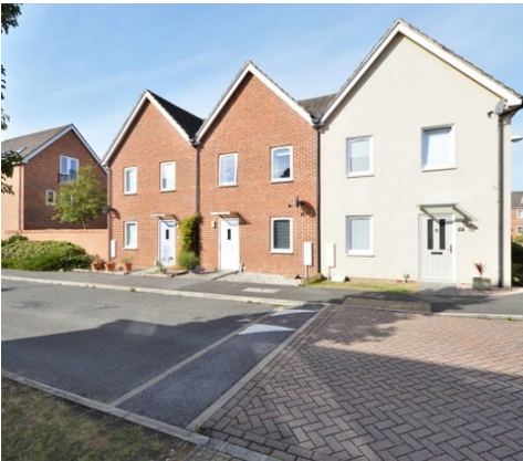
Block sett paving to junction: Tertiary
