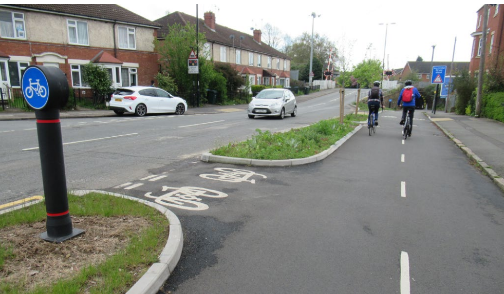
Coventry- segregated cycle track with crossing (image courtesy of WCC)
