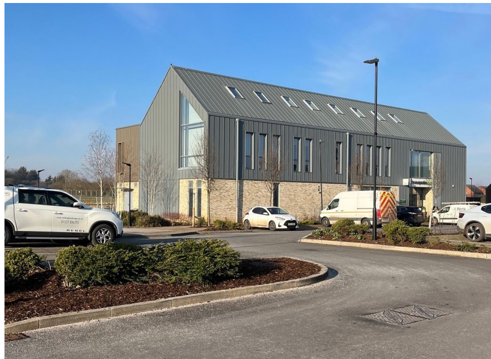
Houlton, Rugby - landscaped car park to mixed use area
