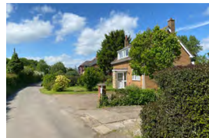
One and a half storey dwelling in a 'traditional' style, finished with buff brick and modern concrete tiles.
