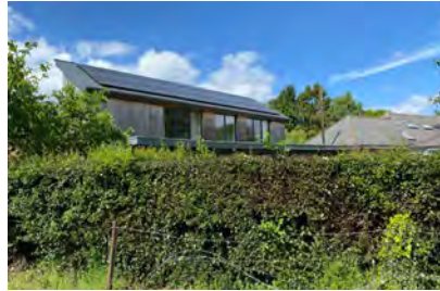
Recent new build two storey dwelling in a contemporary style, using timber as a main facing material and solar panels on the mono pitched roof.
