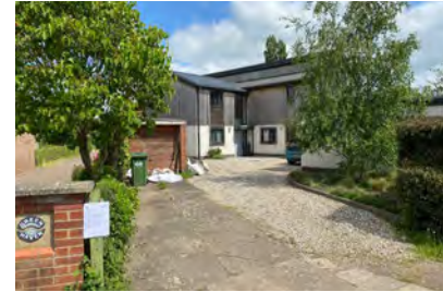
A recent new build two storey dwelling in a contemporary appearance, using timber and off white cement render.
