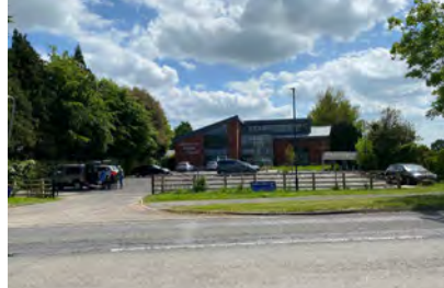
Dunchurch Baptist Church is a two storey building built in a contemporary style, with a mono-pitched roof and faced with red brick and curtain wall glazing.
