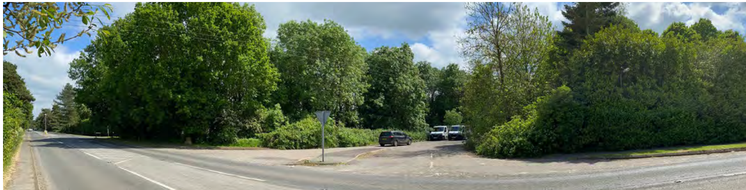
4: Junction of Coventry Road (B4422) and Severn Trent Water Emergency Access Road
