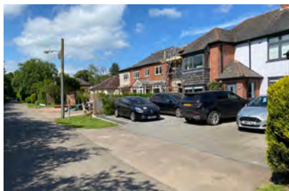
Two storey dwellings with recent additions, mostly finished with red brick and render with roofs covered with slates.
