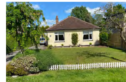
A dwelling with a 'traditional' character, with walls finished with painted render. The single storey bungalow has a hipped roof covered with plain clay tiles.
