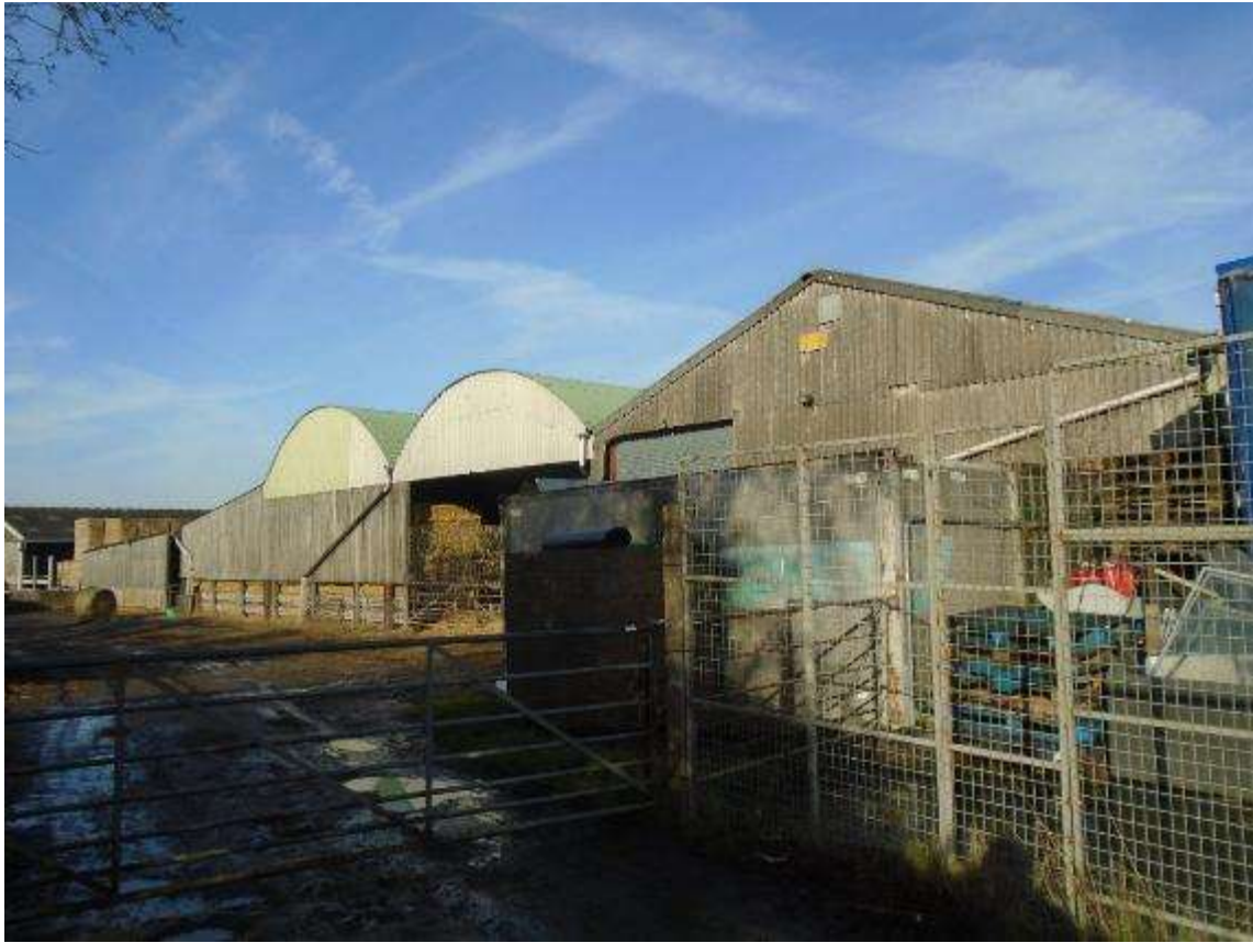
View of the site from the gate located at its southeastern corner.
