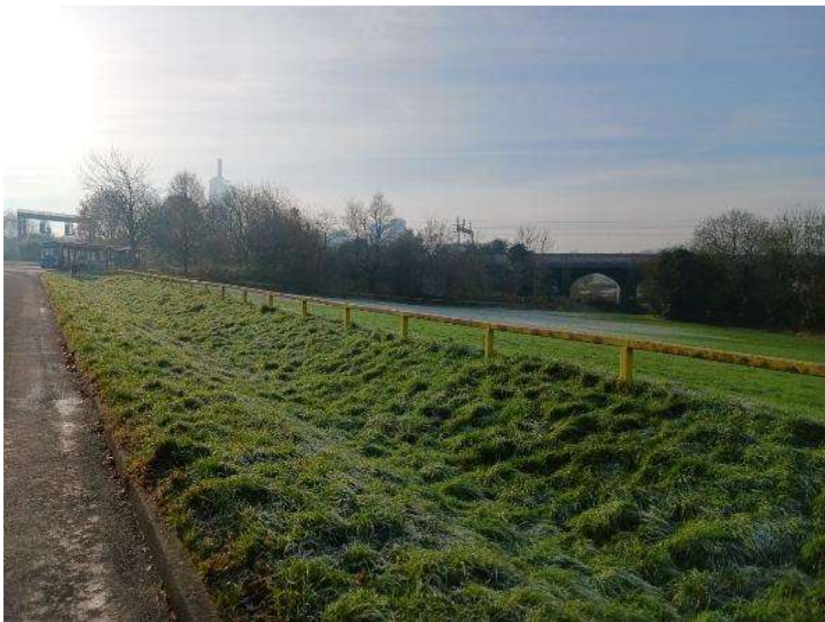
View from the north- eastern edge of the site looking south. Rugby Cement Works visible over the top of the trees.
