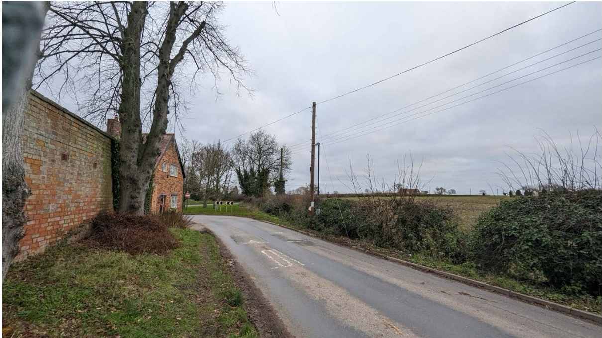
The western boundary of the site (right hand side), which is immediately adjacent to The Old Hall (far ground on the left hand side).
