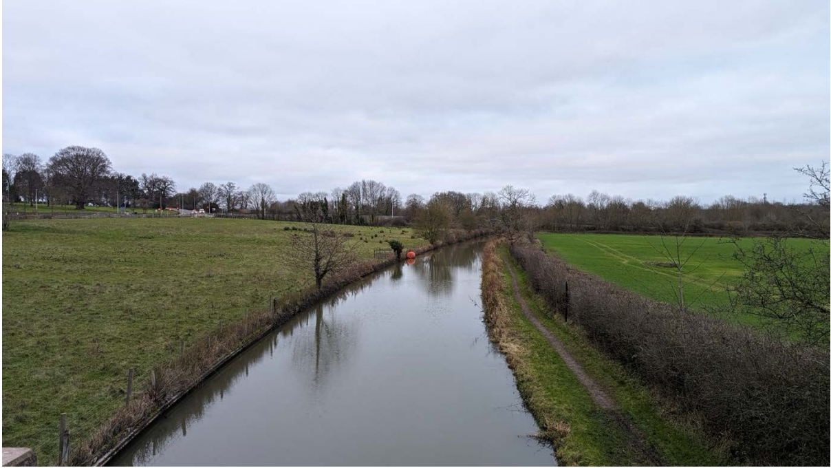
The Oxford Canal and its towpath which runs across the north-western boundary of the site.
