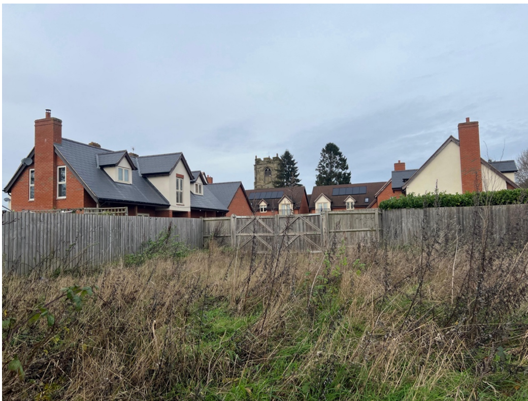
The setting of the church has already changed substantially, with the construction of nearby modern housing.
