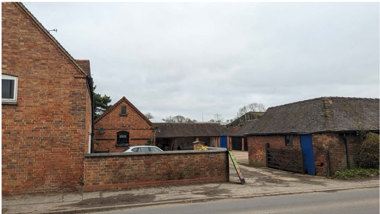
The listed farmhouse and its surviving courtyard buildings.
