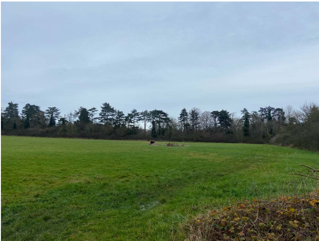
The clearly designed historic boundary of Dunchurch Lodge bounds the site to the north-east and screens the site from views.
