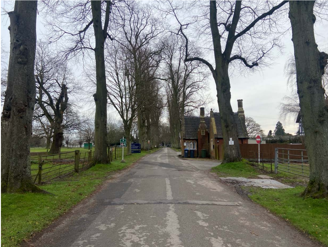
Approach to Bilton Grange along the tree-lined avenue of The Drive. The site is located to the left of this photograph.
