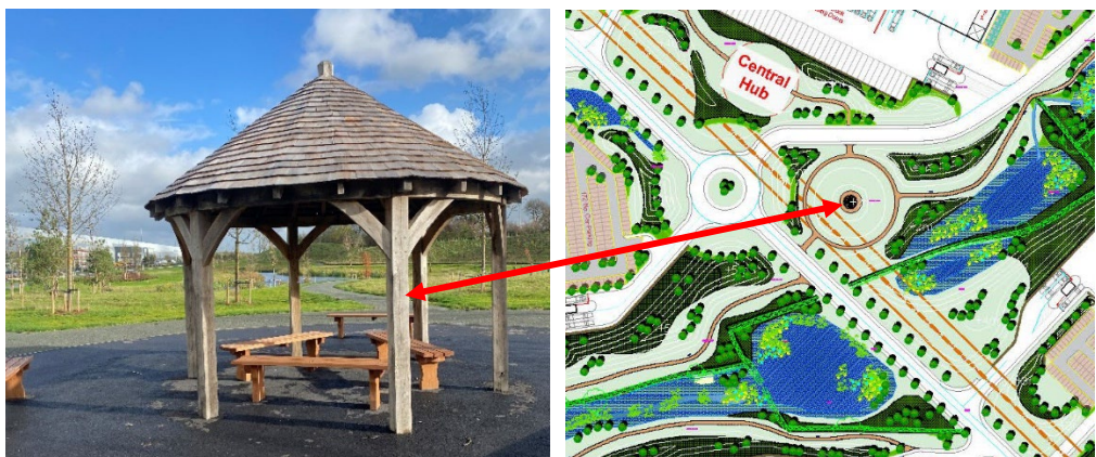
Landscape features set within the Green Blue infrastructure to provide formal and informal recreation along with a sense of place.
