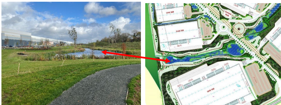
Blue Green infrastructure with plots set within the landscape and by using suitable materials allows access by all abilities throughout the year.
