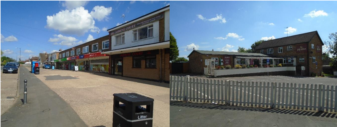
Left: The row of shops on Lower Hillmorton Road with a wide section of concrete hardstanding at their front.
