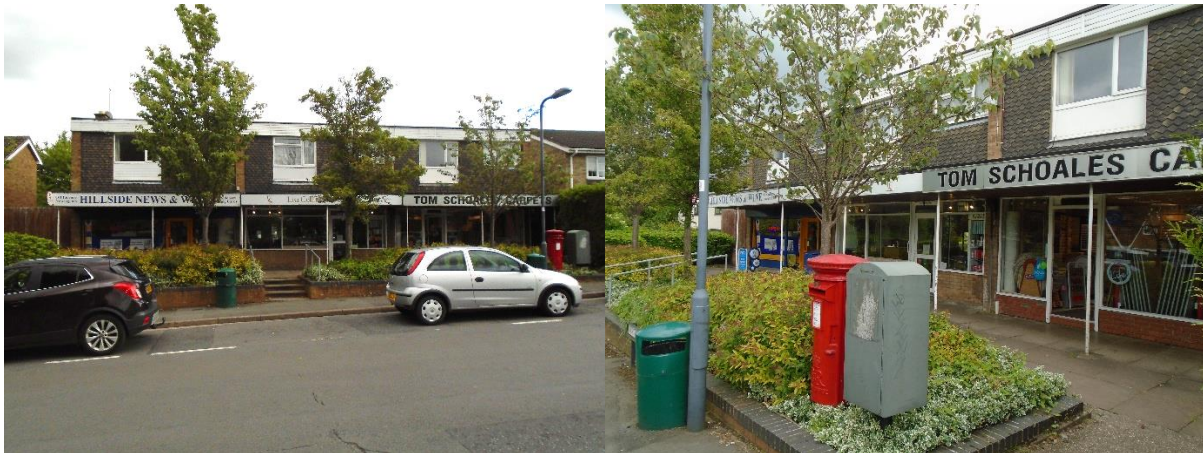
Left and right: The three units that compose the proposed centre, separated from the road by shrubs and trees.
