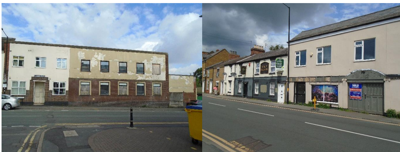
Figure 10 (left): A large vacancy at 135 Railway Terrace, to the north of the residential flats at Lennon Court.
